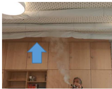
Fig. 11 Porous textile tubes at the ceiling collect the particles
