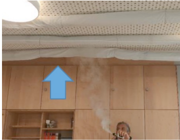
Vertical laminar ventilation to the safe spot over head
